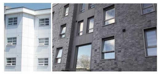
Figure #14-1: Examples of restricted window openings; (left): Only one of six panes was openable, and only to a limited extent - the flats overheated (GHA Preventing overheating report, 2014); right: only the top  $\frac{2}{3}$  part of windows opens, and the opening is restricted to only a very small gap.
