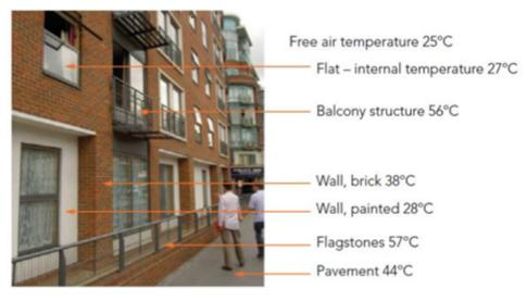
Figure 9-1: A study carried out by the BRE showed that surface temperatures contributed to overheating risk, with south-facing exposed brick facades and tarmac areas nearby contributing to high temperatures near air inlets.
