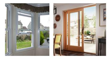
Figure #14-2: Examples of openings providing just under 50% free area: window with bottom half opening; patio door
