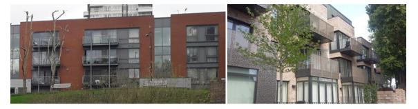
Figure #13-2: Examples of shading from balconies. On the right-hand side example, proportions of glazing are lower and shading more comprehensive. On the left hand-side, the building is highly glazed (around 65%, and a fully glazed circulation area), shading is only partial as a number glazed areas have none. In both cases, the top floor apartments have no balconies above and are therefore more exposed to solar gains.
