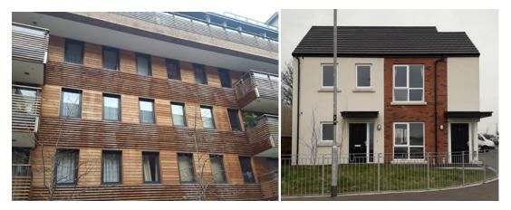
Figure #6-2: Example of glazing proportion between 35% and 50% of facade area
