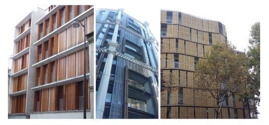
Figure #13-1: Examples of movable shading devices. They are used differently across the facade, showing user adaptation.
